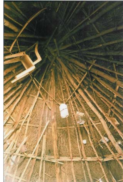
Building Construction. Fig. 9 Simple Bungha roof from the inside (photo by the author).
